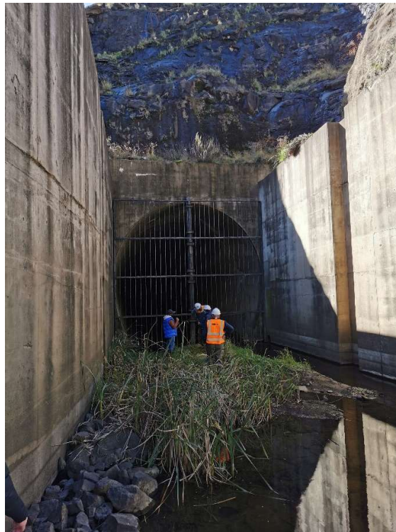
Figure 3: Diversion Tunnel No.2 Portal
